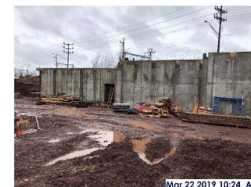
Mar 22 2019 10:24 AM Form work stripped at north foundation walls
