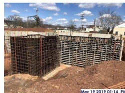
Mar 19 2019 01:14 PM Form work for foundation walls at main entrance
