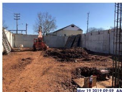
Mar 19 2019 09:59 AM Foundation walls complete at southeast corner
